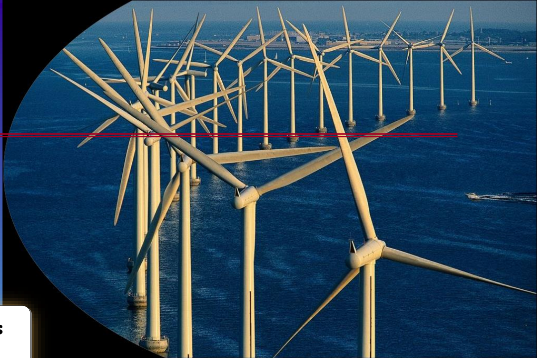
Middelgrunden offshore wind farm, near Copenhagen, Denmark (55°40' N, 12°38' E). http://www.yannarthusbertrand.org
